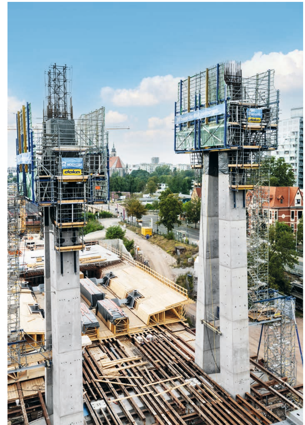
2 Safe working even at great heights thanks to self-climbing formwork and all-round enclosure.
