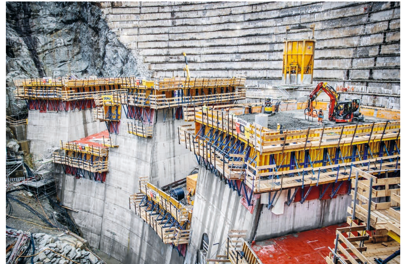
2 The Grimsel consortium is using Doka's formwork solutions and digital services.
