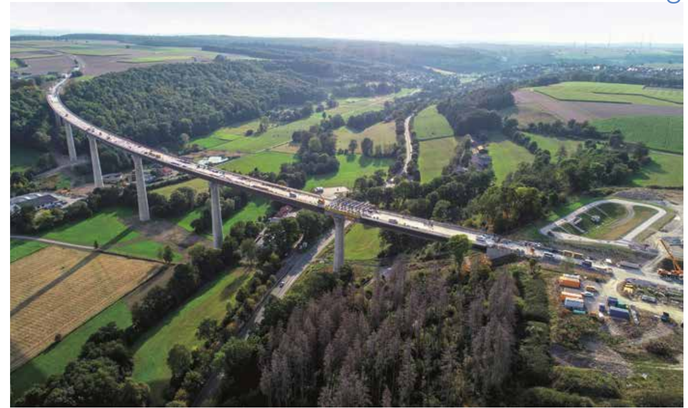
1 After a construction period of six years, the 785 metre long Aftetal bridge will be opened to traffic in spring 2022.
