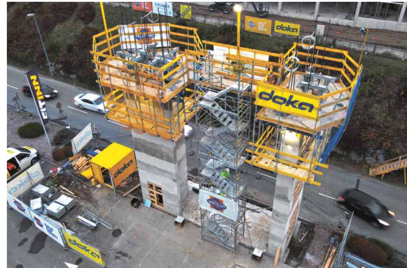
1 Successful first use of Doka-Slipform when constructing a staircase.
