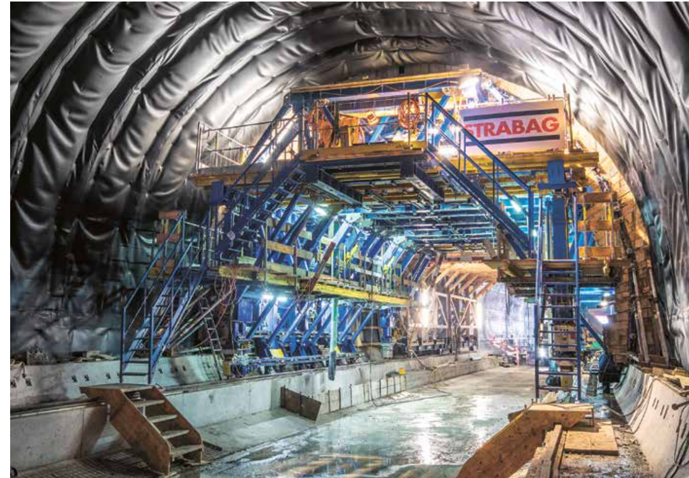
1 Generous access openings ensure smooth construction site traffic.
