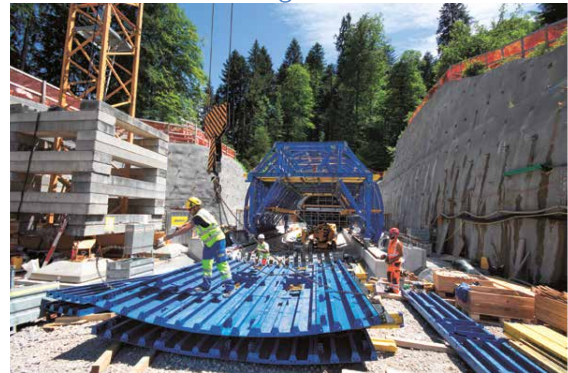
2 Rapid progress on site thanks to pre-assembled and ready-to-use formwork components.
