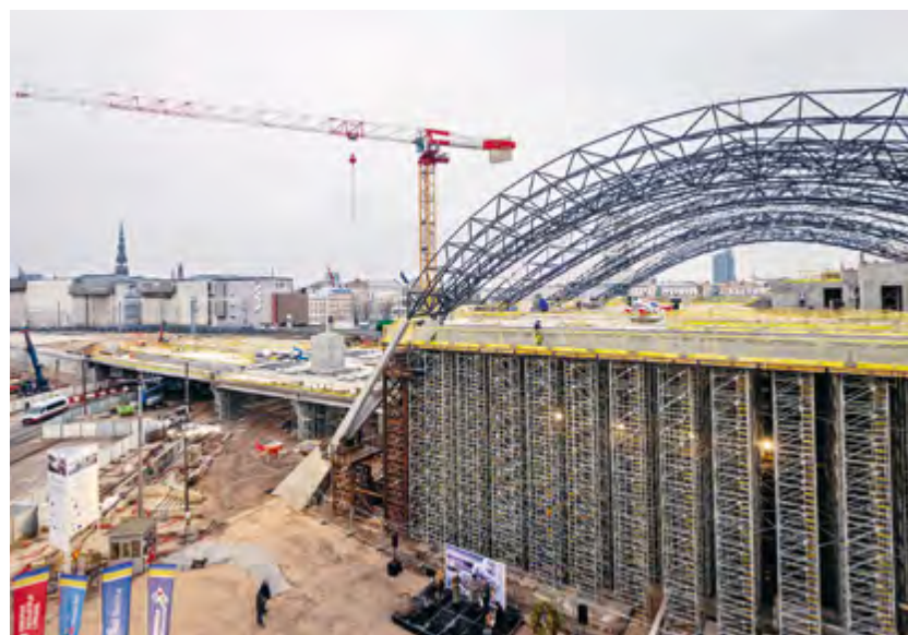
For the construction of the bridge to and from the railway station, Doka Staxo and Ringlock were used, as well as the Concremote concrete monitoring system.
