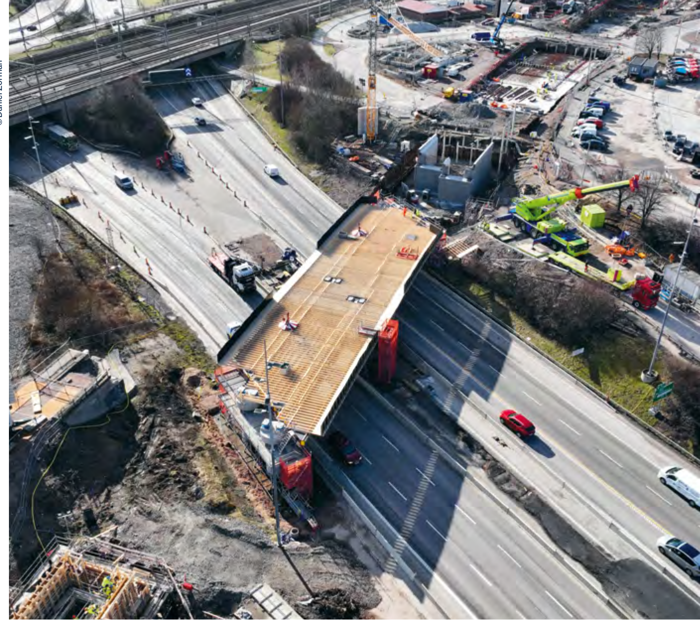
Spans of up to 22 metres have to be bridged to keep traffic flowing despite the construction work.
