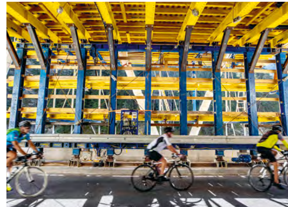
Doka UniKit – the universal engineering kit for heavy loads – provides unrestricted traffic clearance.
