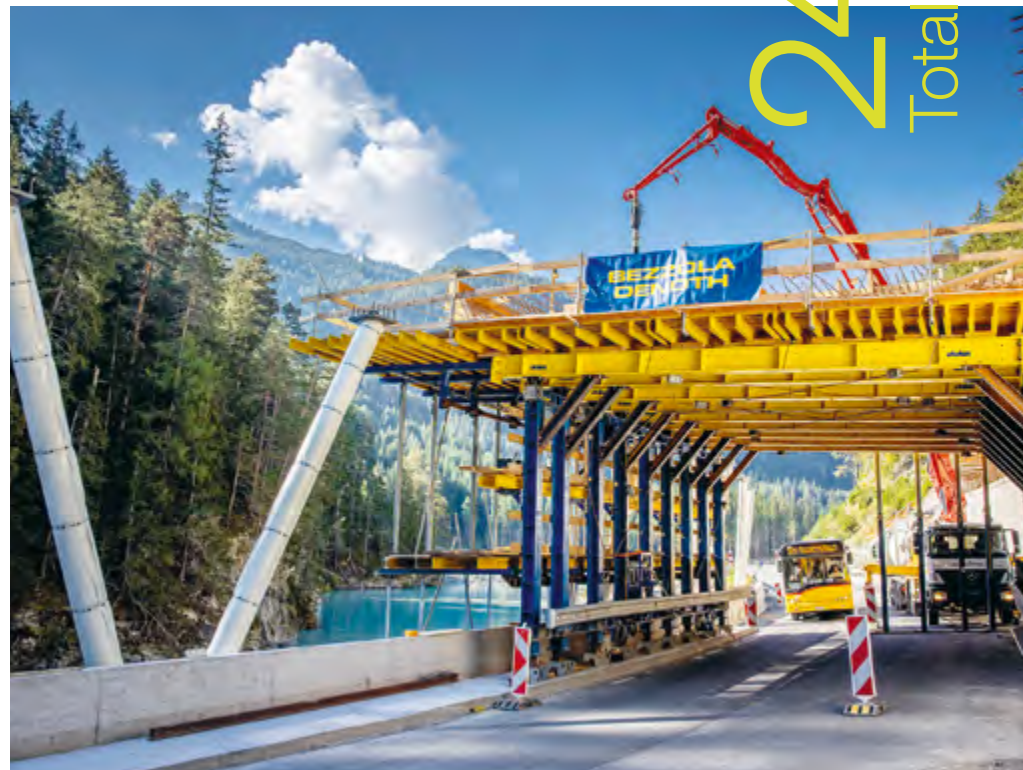
Doka UniKit – the universal engineering kit for heavy loads – provides unrestricted traffic clearance.
