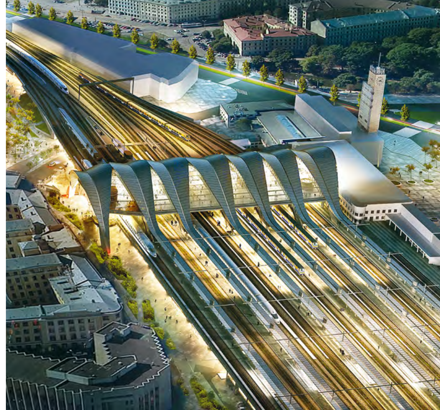
Riga Central Railway Hub will become the largest passenger terminal in the Baltics.
