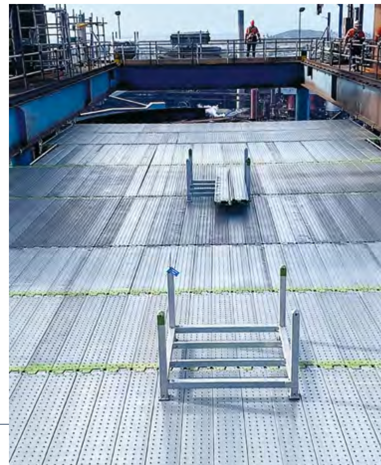
The team created Australia's largest suspended work platform using the Ringlock Raised Ledger system.
